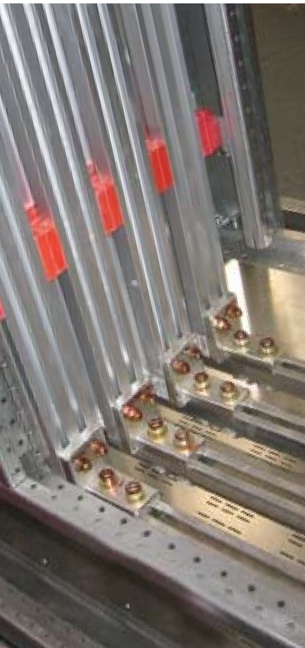
Cast copper connection on main Busbars to distribution bars
