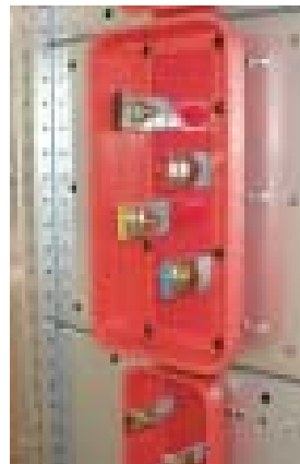
Outgoing terminals with boot retainer
