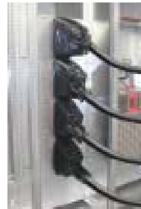
Flexible boots fitted to retainer Form 4b Type 5
