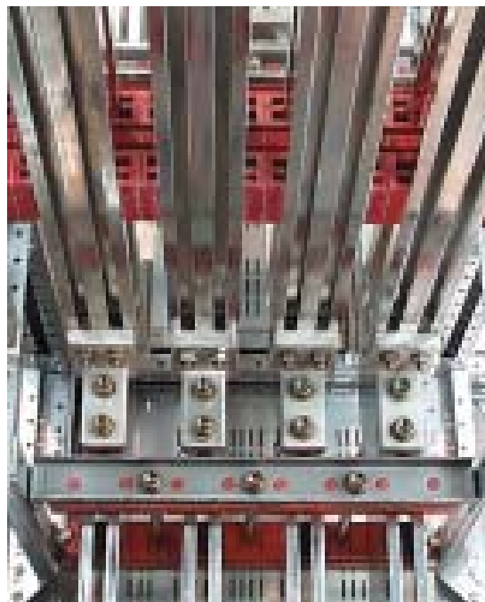
Cast copper connection on main Busbars to distribution bars
