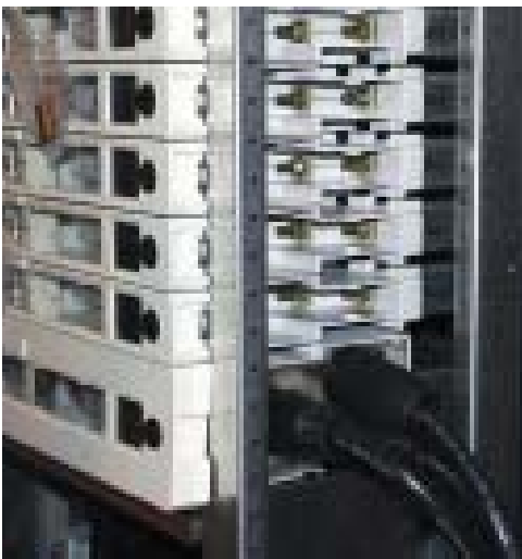
Slimline Switchfuse with outgoing cables
