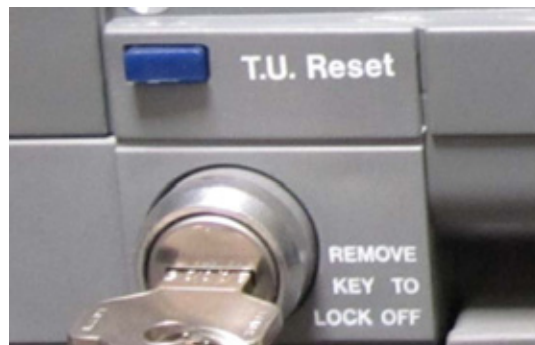
Emax V2 - PR121/P - The normal position of the trip reset button
