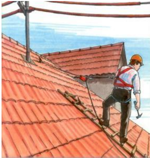
Working on roof ladder fixed on roof plane
