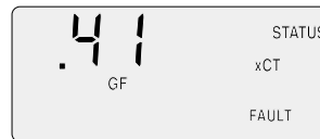
Breaker tripped on ground fault
