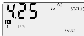
Breaker tripped on long time
